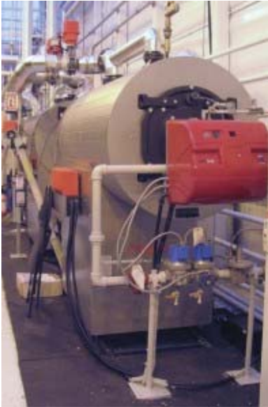
Condensing boiler
